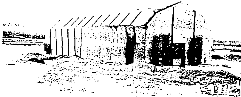
Fig. B.15 — Structure 3.13b Prior to Shot 9.
